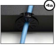
Wrap the split grommets around the cables and insert the grommets back into the holes in the Rack Tray.
